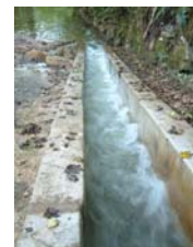
Impassable barriers fragment habitat, obstruct migration and prevent re-colonisation of species after pollution events. Here a fish pass has been installed to reconnect and open up valuable habitat.
