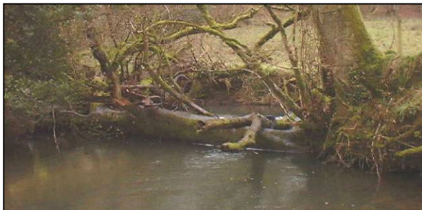
A fallen tree may cause a blockage that will result in erosion
